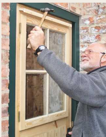
▲ Pic.5 ...and it the weather moulding with screws that are hidden by pellets
